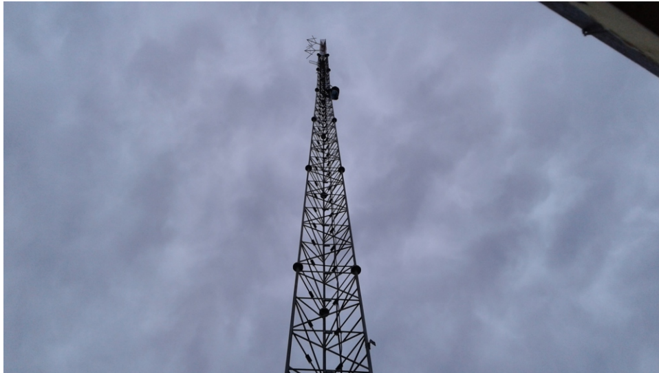
Figure 7: Eric Duncan, tower rigger with Duncan & Sons, ascending tower in order to realign the azimuth of the STL antenna in order to peak the received STL signal level.
